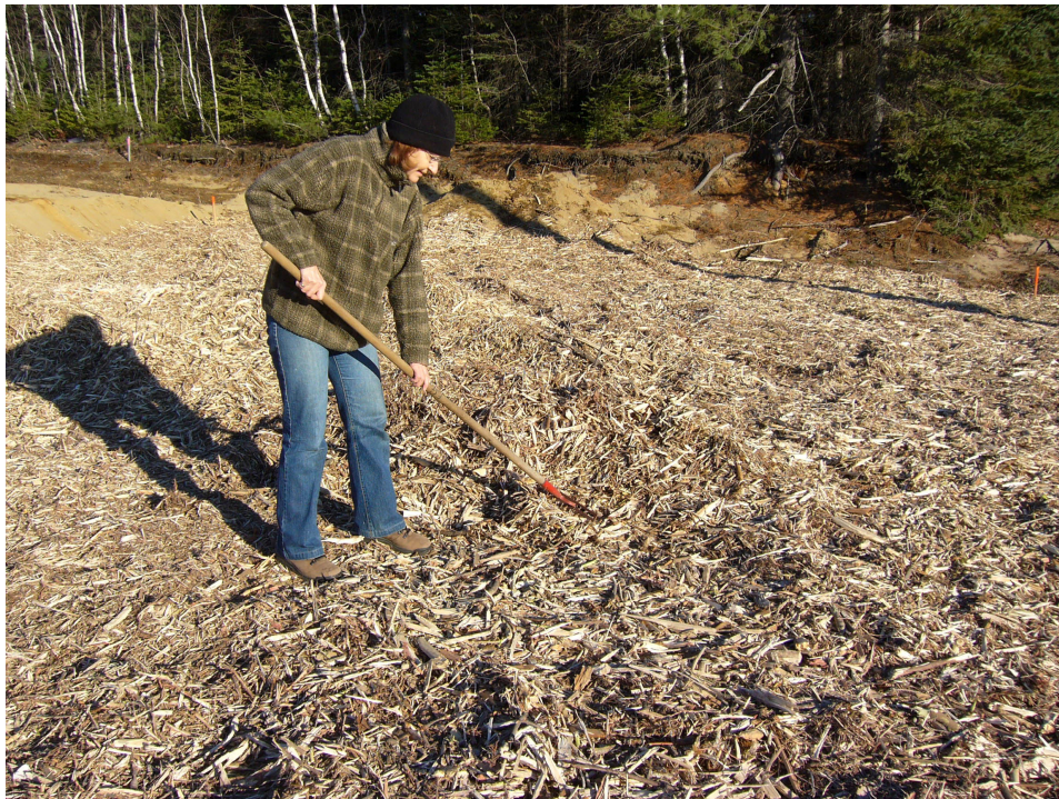
Figure 5. Spreading RCW with a rake
